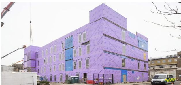
Fig.5 Hospital Construction site
